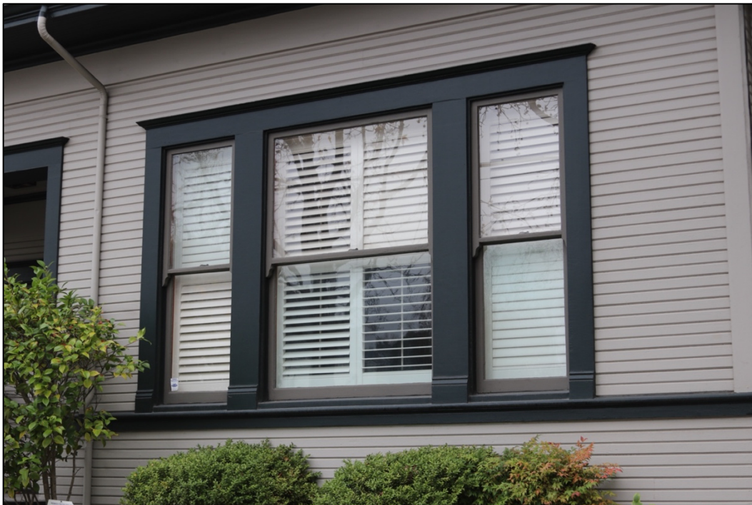
Figure 2: West elevation, tripartite windows
