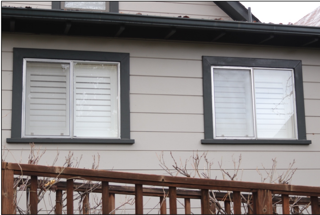
Figure 27: East elevation, modern aluminum sliding windows
