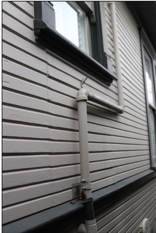
Figure 12: North elevation, patched siding (possible window infill)
