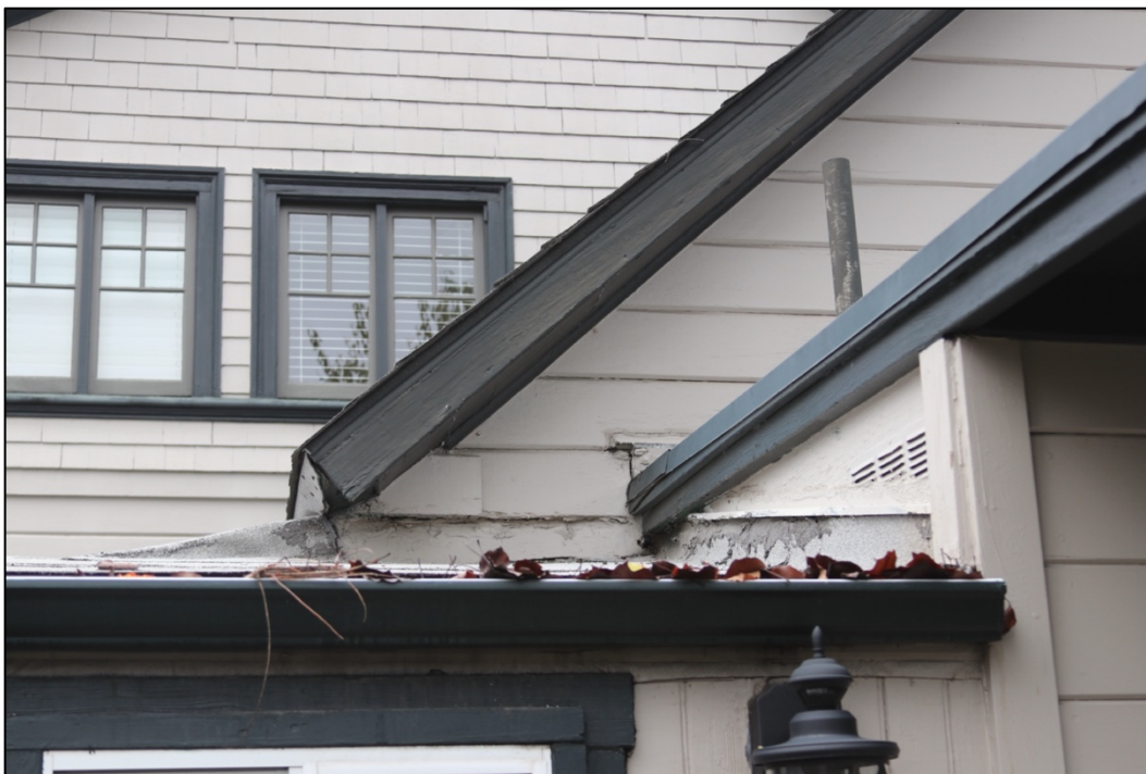
Figure 25: East elevation, fascia boards
