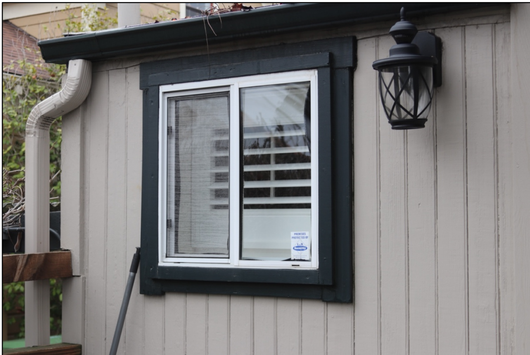
Figure 28: East elevation, modern aluminum sliding window
